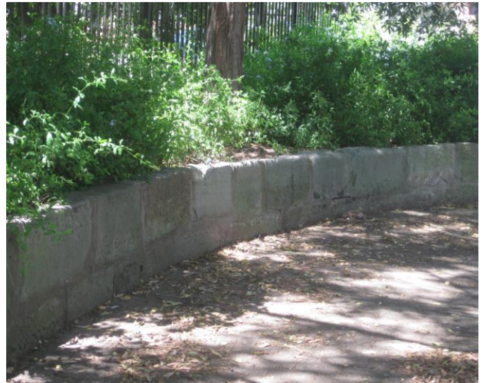
Ibrox Park formerly Derbyshire Reserve (3), 2015 Curved Sandstone Block Wall, Garden, Paving Adjacent to Sydney Secondary College
